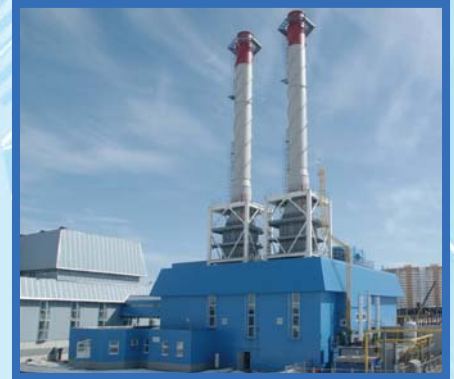
Gas-turbine electric power unit with the capacity of 10 MW
