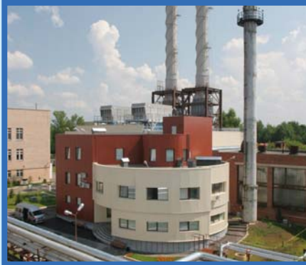
Gas-turbine electric power unit with the capacity of 6 MW
