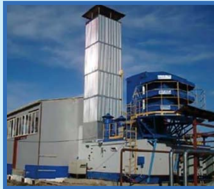
Gas-pumping unit with the capacity of 4 MW
