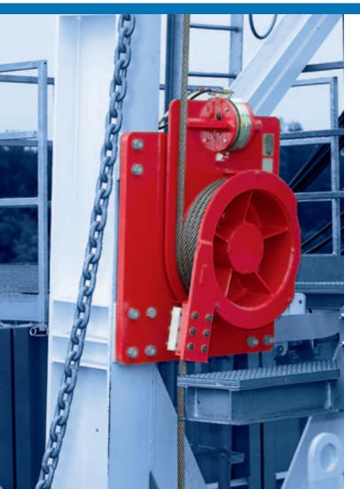
Designed to be used with compression load cells, the Bentec DEADLINE ANCHORS are made from high-grade structural steel for operation in harsh work environments from -40°C up to +55°C.
